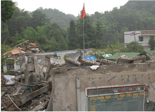
Collapsed teaching building
