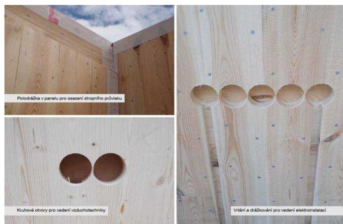
Obr.15-CLT deska s vruty(pohled) (DEKPANEL, © 2022)
