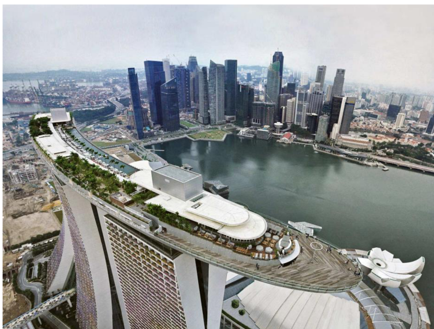
Obr. 9 Zahrada Marina Bay Sands Rooftop Garden (Green Roofs, Marina Bay Sands Integrated Resort Skypark ©2022)
