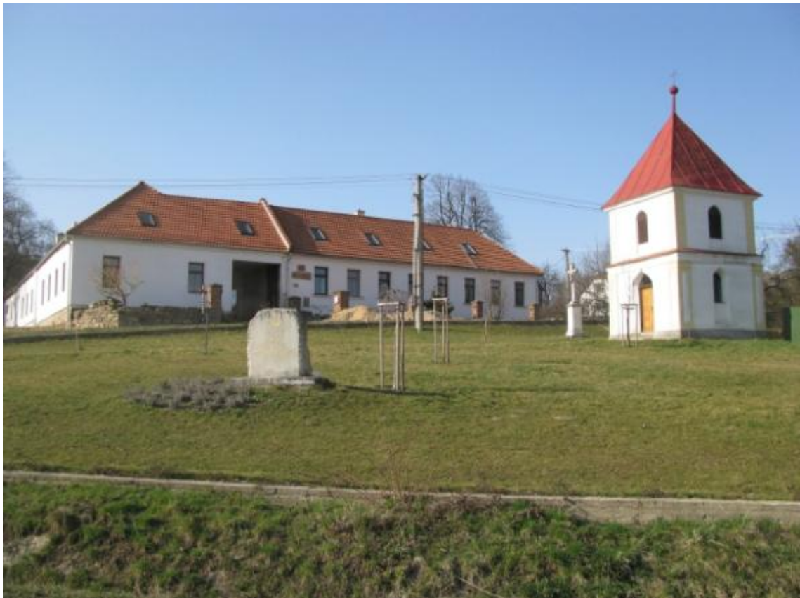
Fig. 1: Building of TC Sejřek. Source: Sobotka J., 2008.
