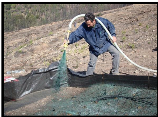
Photo 34. Manual application of hydromulch at the controlled area (Ferreira, 2014).
