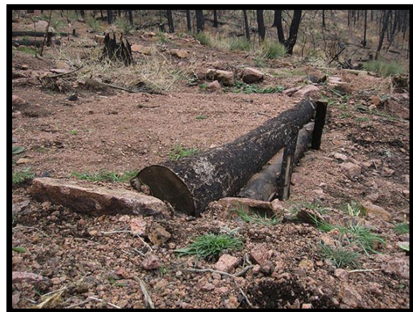
Photo 38. Log barrier fitted in the terrain as a antierosion measure (www.markitforestry.com).
