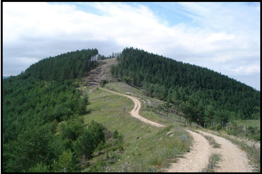
Photo 27. Example of strategic fire break between two production sites with forest road in the middle for better access for firemen in case of fire threat, in this case as in the many existing the width is less than 100 m (www.navarra.es)
