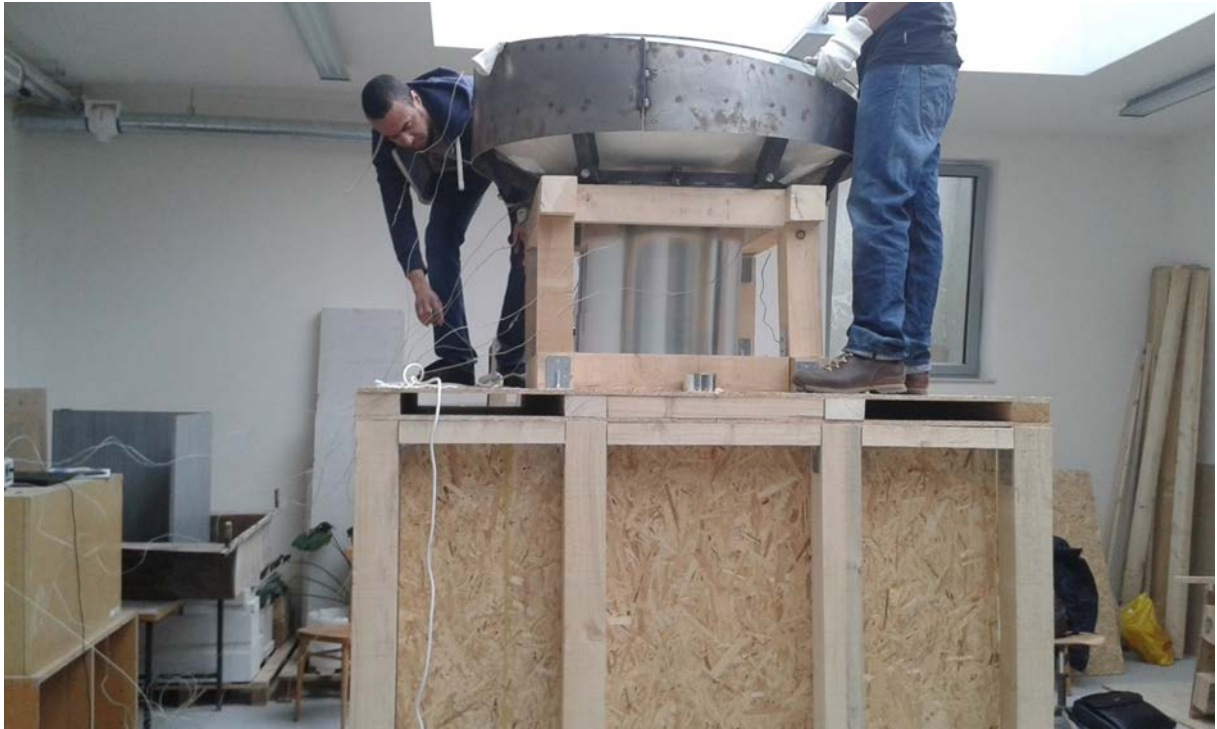
Fig. 3.9: Construction of CH1
