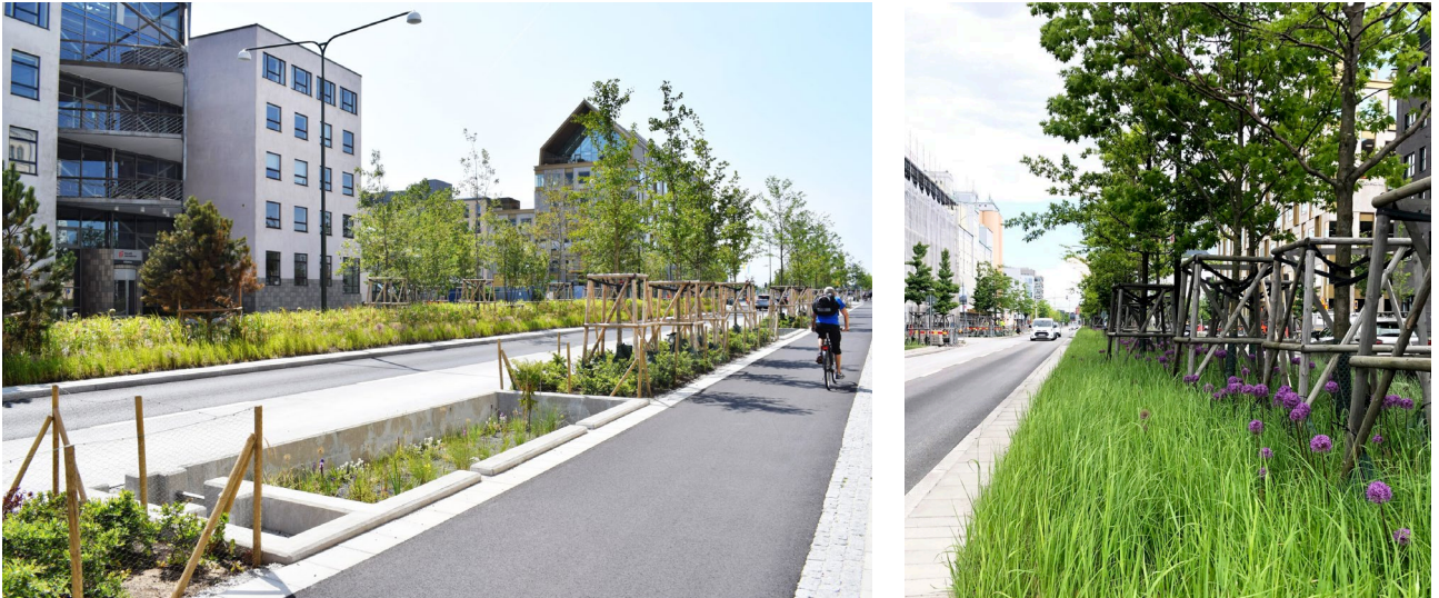
Pic. 6 The rain garden collects water from the surroundings. The excess is regulated and discharged into the storm drain. Pic. 7 Vegetation fragment.
