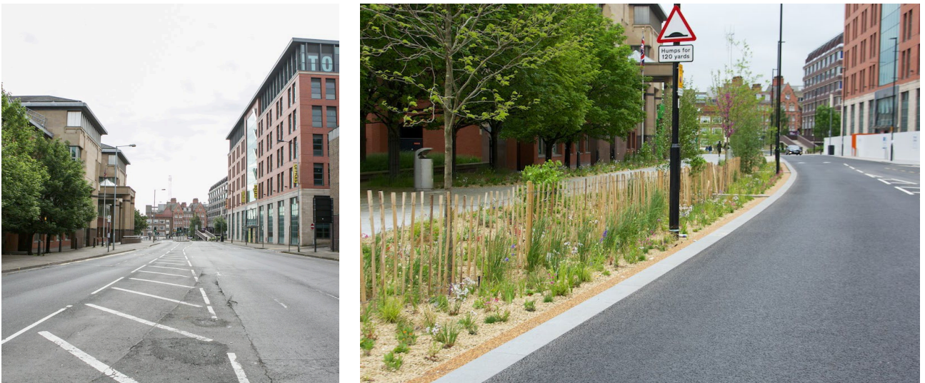
Pic. 8 Site before the grey to green transformation. Pic. 9 Site after transformation. Water from adjacent surfaces is drained to the rain gardens and bioswales.
