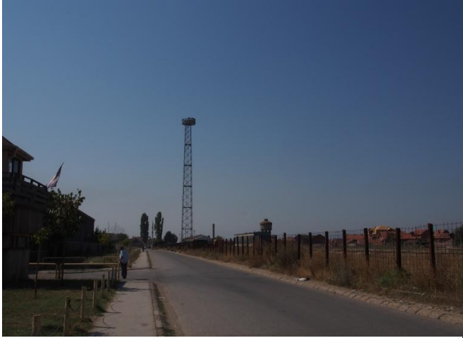
Picture 5 The road connecting railway station to neighbourhoods 28 and 29
