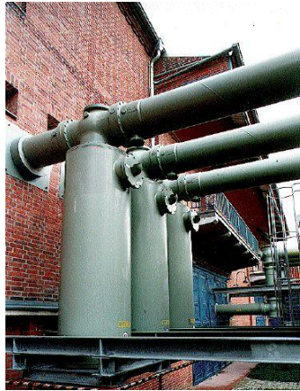
Fig. 3-23: Typical installation of a GIS arrester. [14]
