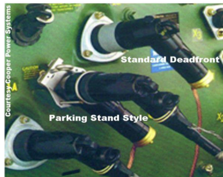
Fig. 3-24: Underground Circuit with Deadfront arrester. [2]
