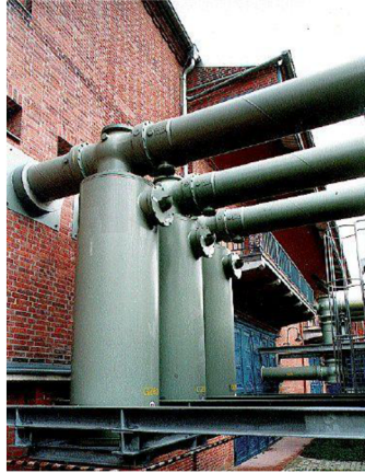
Fig. 3-23: Typical installation of a GIS arrester. [14]
