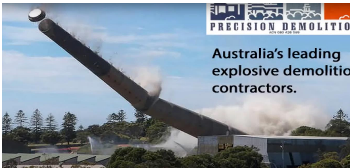
Obrázek 14: Swan Bank Chimney Demolition, https://www.youtube.com/watch?v=iXPipFq1HA8 [24]
