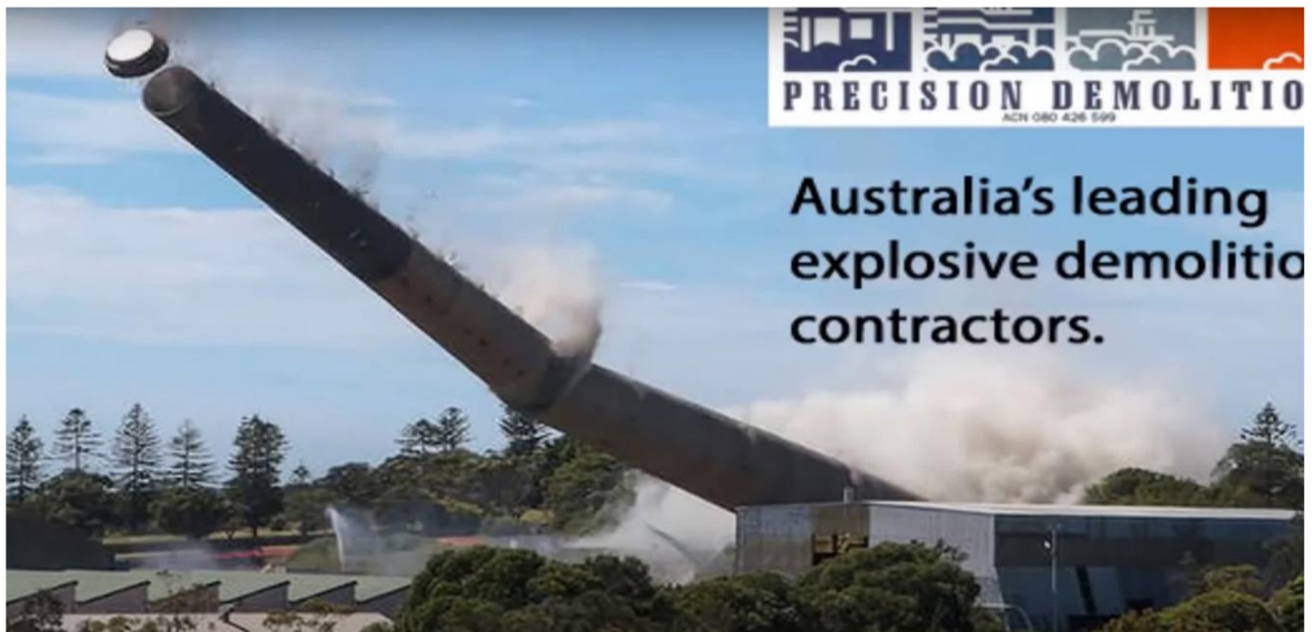
Obrázek 14: Swan Bank Chimney Demolition, https://www.youtube.com/watch?v=iXPipFq1HA8 [24]
