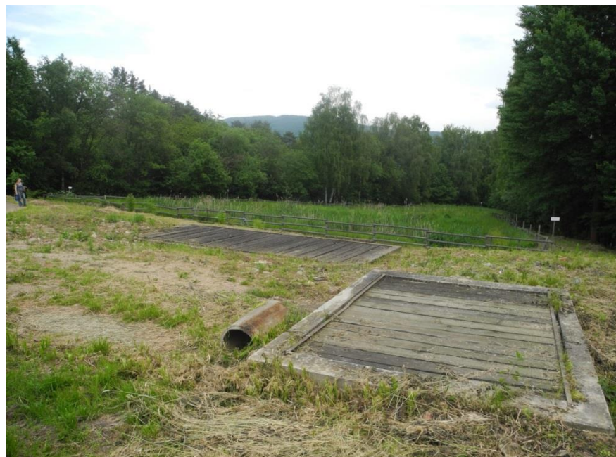
Figure 4: Overview of the constructed wetlands.
