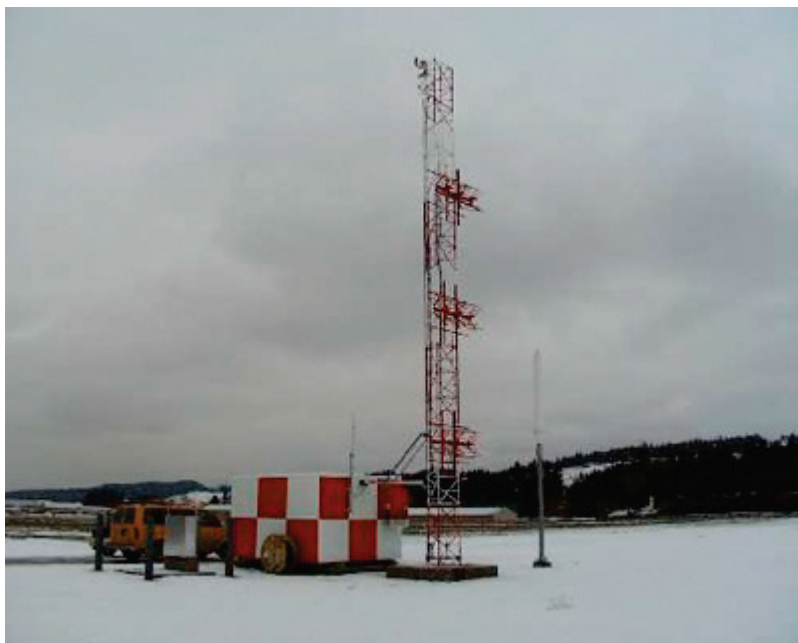
Obr. 2 GP anténa [www.navcanada.ca]
