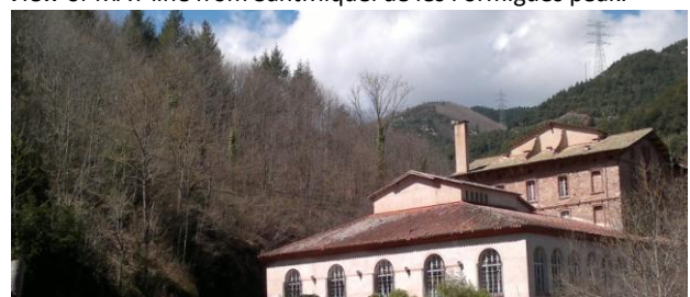
MAT line crossing Osor's brook on Font Picant place.
