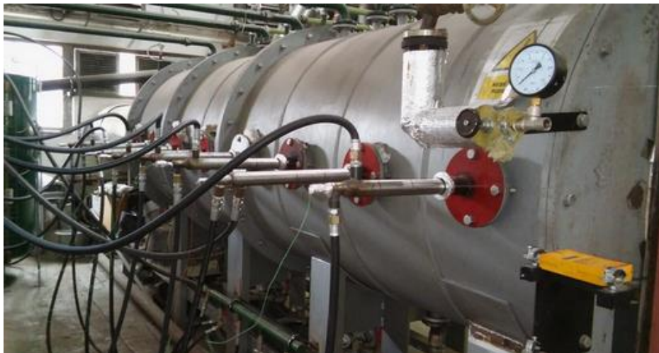
Fig. 26: Detail of thermocouples for measuring temperatures in the combustion chamber
