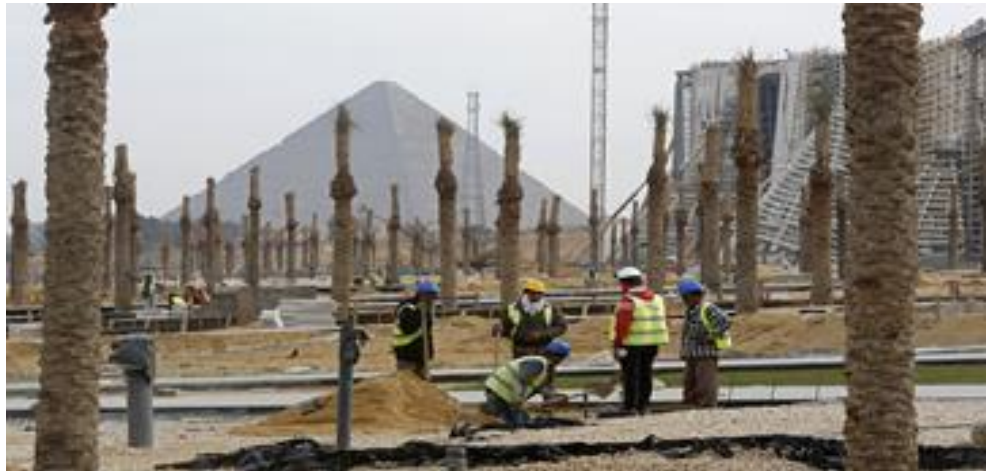
Figure 8 Construction in Egypt
