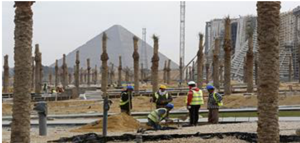
Figure 8 Construction in Egypt
