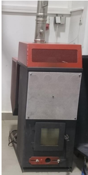
Figure 16. Automatic pellet boiler (Source: Author, 2017)
