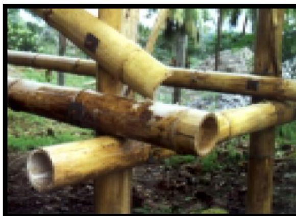
Fig. 64: A joint in Group 5, with steel bolts
