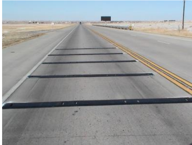
Figure 2.8 Example of temporary rumble strips
