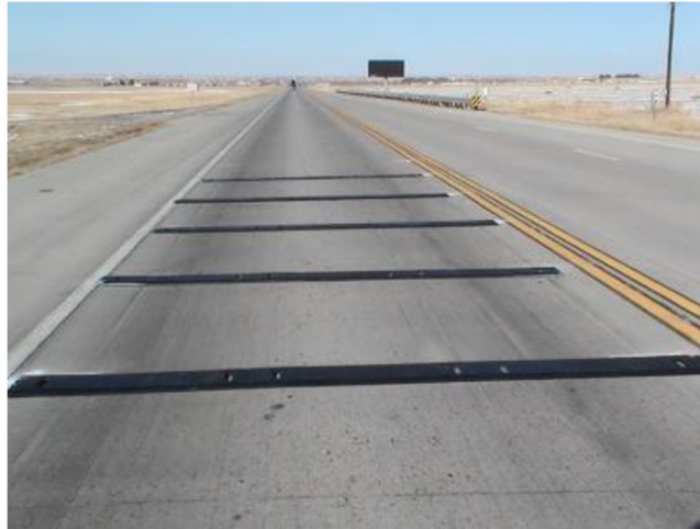
Figure 2.8 Example of temporary rumble strips
