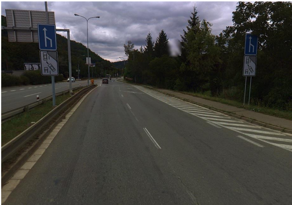
Figure 3.1 Detail of the lane merging in Brno. The end of the on-ramp can be seen in bottom right.
