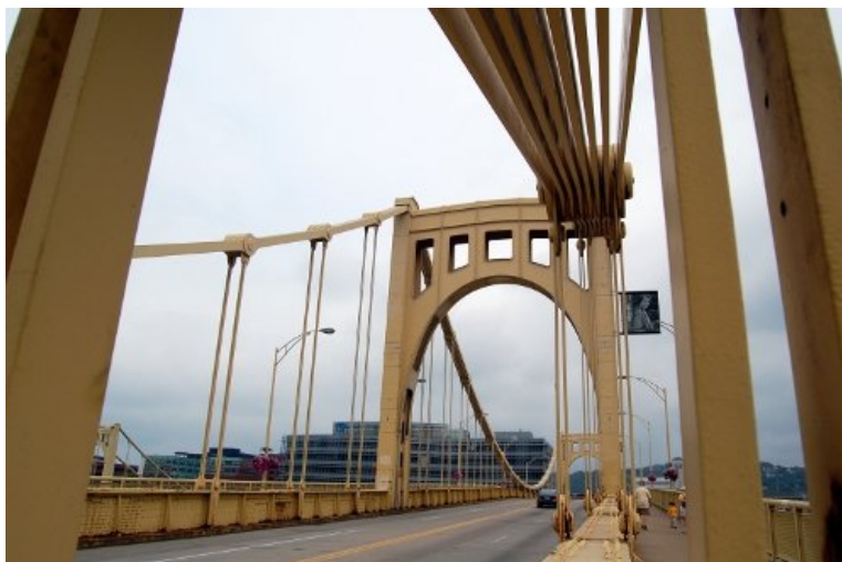
Obr. 4 Visutý most Three Sister's Bridge, Pittsburgh – multiparalelní „eyebar” systém [2]
