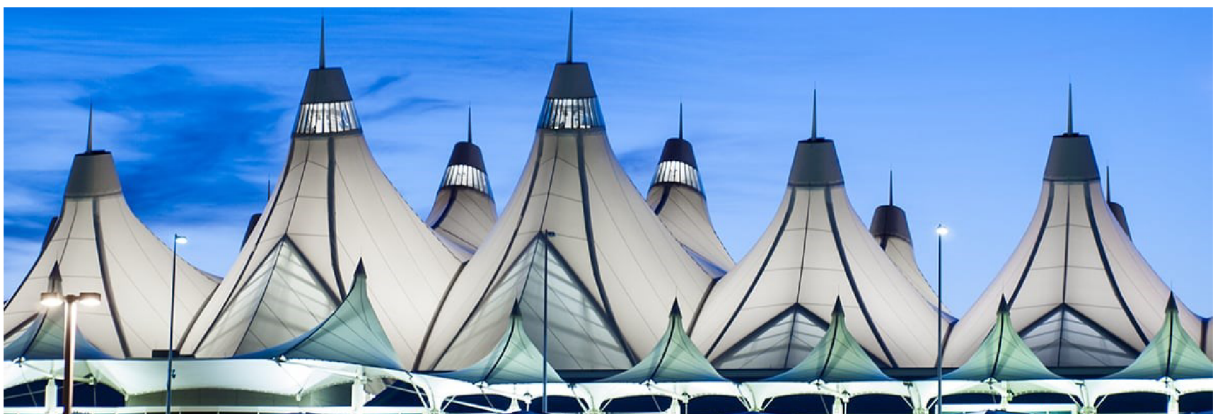
Fig. 2 Roof of Denver International Airport, USA [III]
