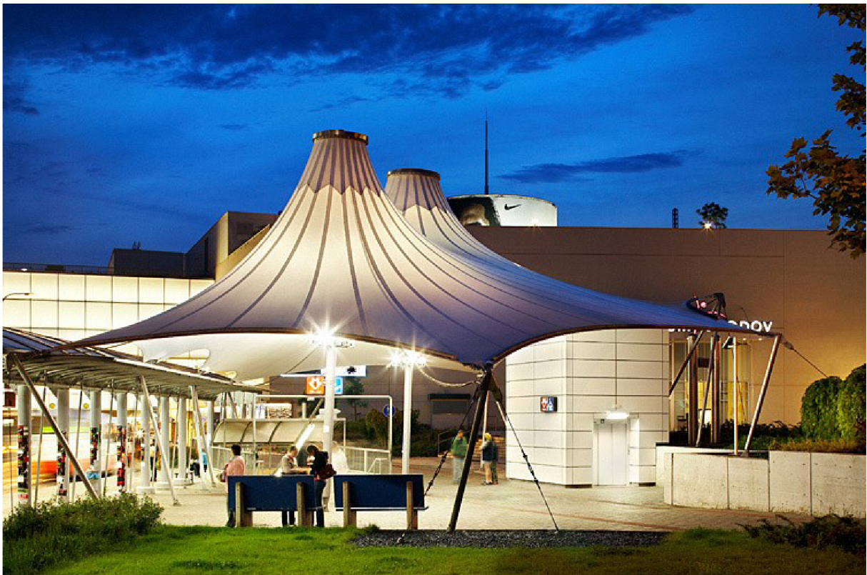
Fig. 143 Shopping Centre Chodov in Prague (East Exit from Metro), Czech Republic [X]
