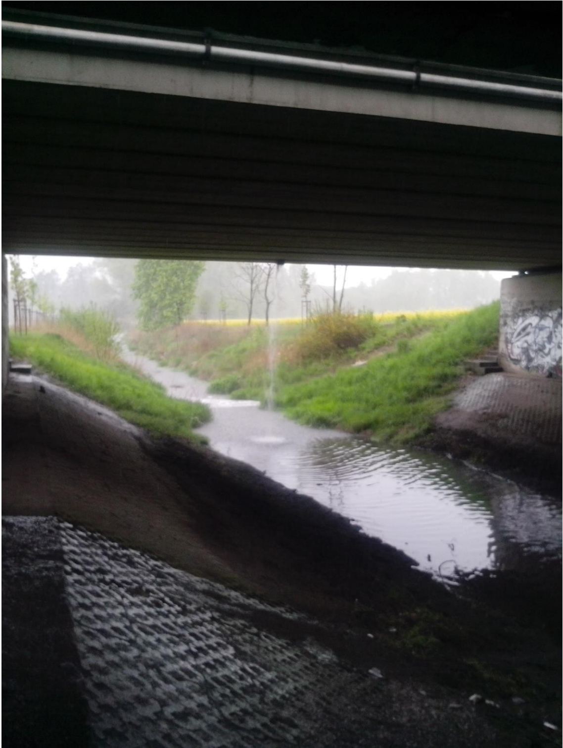
Fig. 20. Highway bridge over Rostěnický stream (D1–267 km), direction towards Vyškov town (28 th April 2016, photo of author)
