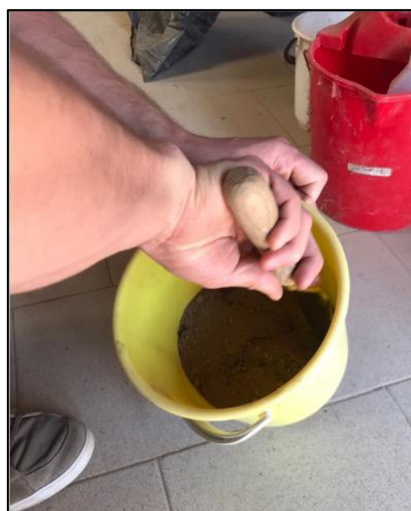
Figure 11 Mixing process in the bucket
