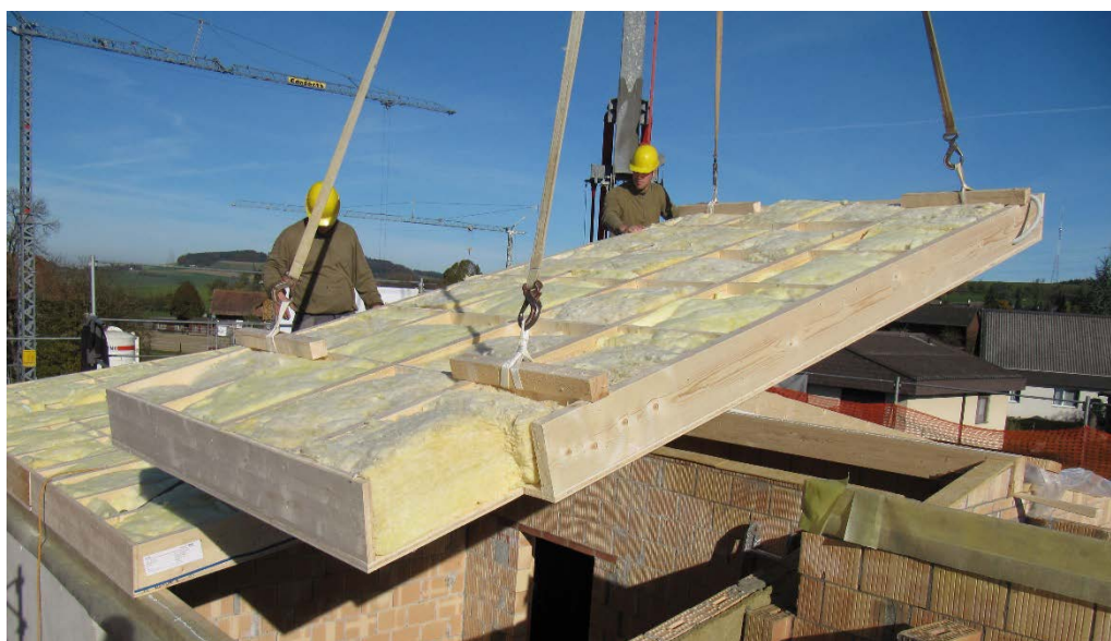
Obr. 12 Montáž MT Open (Agrop Nova, 2017)
