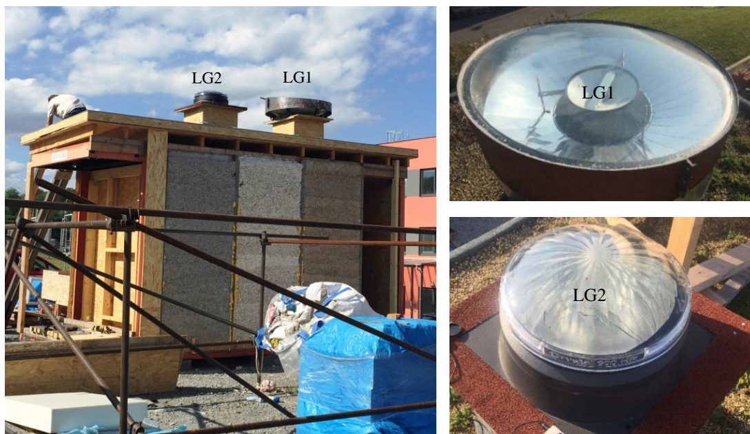
Fig. 4.4: Tested light guides LG1 and LG2 – the roof installation
