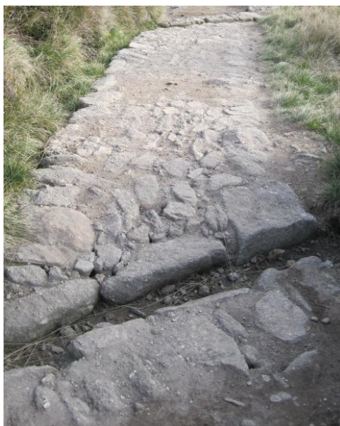
Figure 8 Reconstructed (left) and old (right) sections of trail through Obří důl (Photo: Author)
