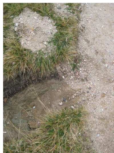
Figure 9 Recently cleaned water bar orifice - Pramen Labe trail (Photo Author)
