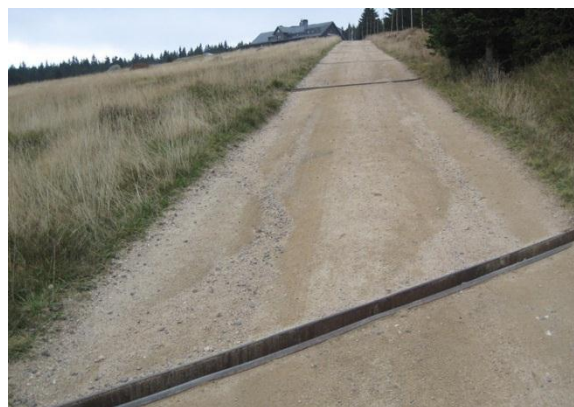
Figure 11 Vosecká trail - ruts with eroded CWGG (Photo: Author)
