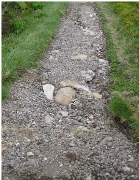
Figure 13 Eroded trail to Jestřábí bouda with alkaline material (Photo: KRNAP)
