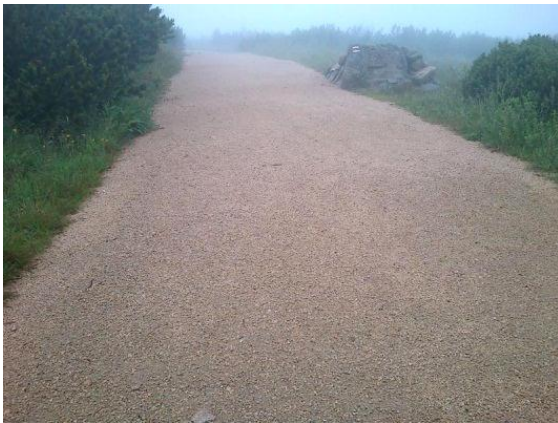
Figure 4 Trail with compacted weathered granite gravel surface (Photo:Author)
