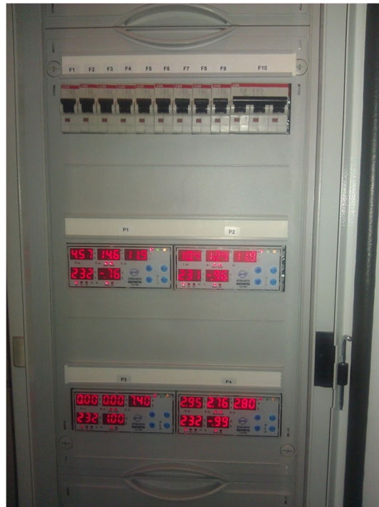
Figure 18 : Current measurement setup (only Instruments shown)
