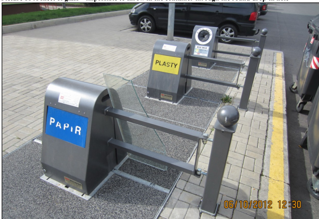
Picture 11 A sheet of glass – impossible to throw in the container through the round drop-in hole
