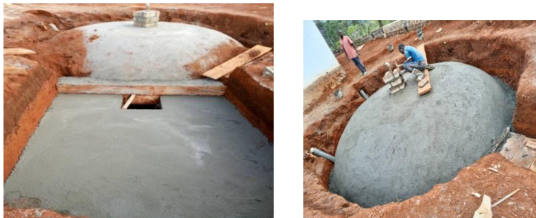
Figure 2: Construction of a 30 m 3 biogas in the mile 4 Nkwen slaughterhouse to be used mainly for cooking.
