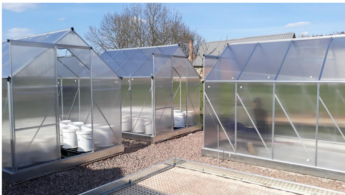
Figure 2: A photograph captures the completion of three out of four experimental greenhouses at the SÚRO complex in Hradec Králové.
