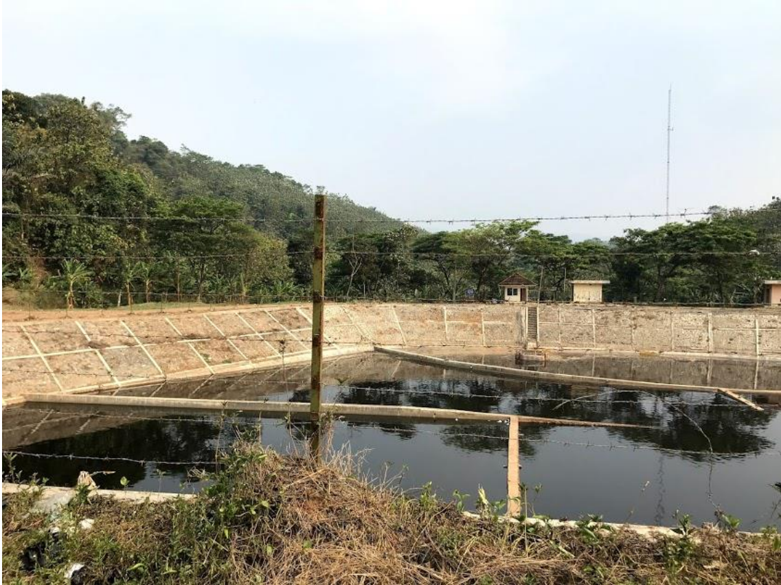
Figure 18.: Leachate collection pond in Sarimukti disposal site (Author 2018).
