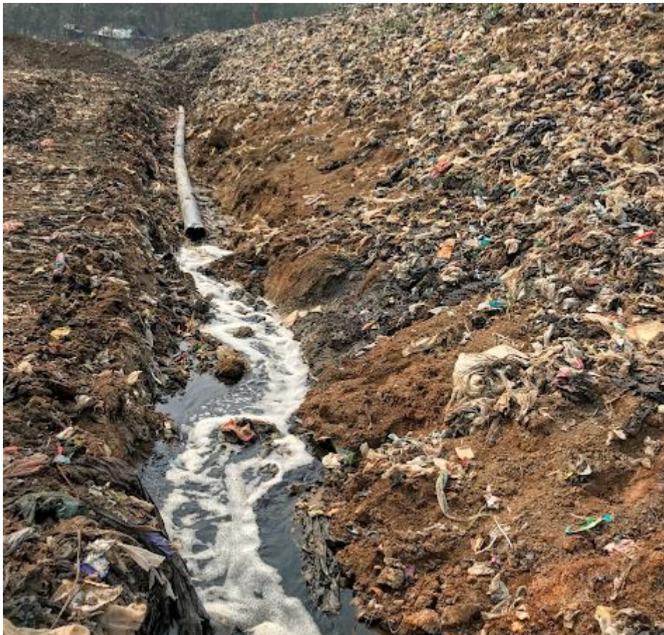
Figure 10.: Leachate collection drainage on Sarimukti disposal site (Author 2018).
