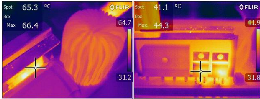
Fig. 82: Thermal camera picture of power stage during operation at full power 3kW – GaN half bridge on insulated metal substrate board (left), synchronous rectifiers (right)
