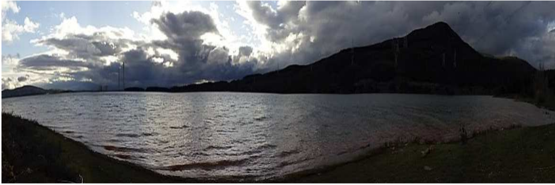
Pic 6. Reservoir Of Barcena with the thermal power plant of Compostilla II. Pablo F. Arias 2014.
