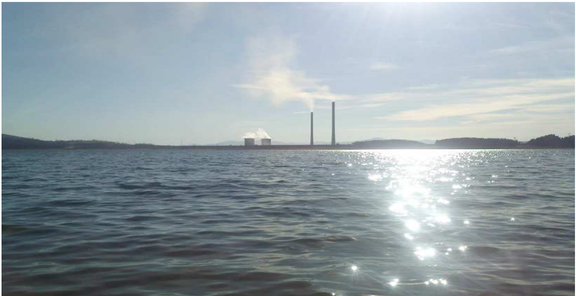
Pic 5. Reservoir Of Barcena with the thermal power plant of Compostilla II. Pablo F. Arias
