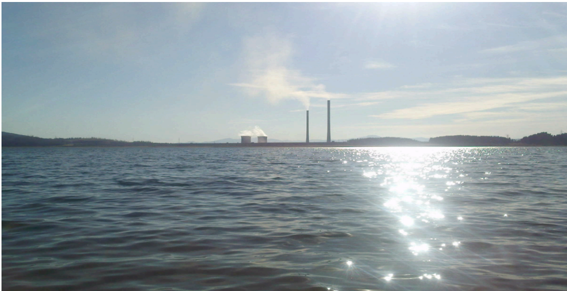
Pic 5. Reservoir Of Barcena with the thermal power plant of Compostilla II. Pablo F. Arias
