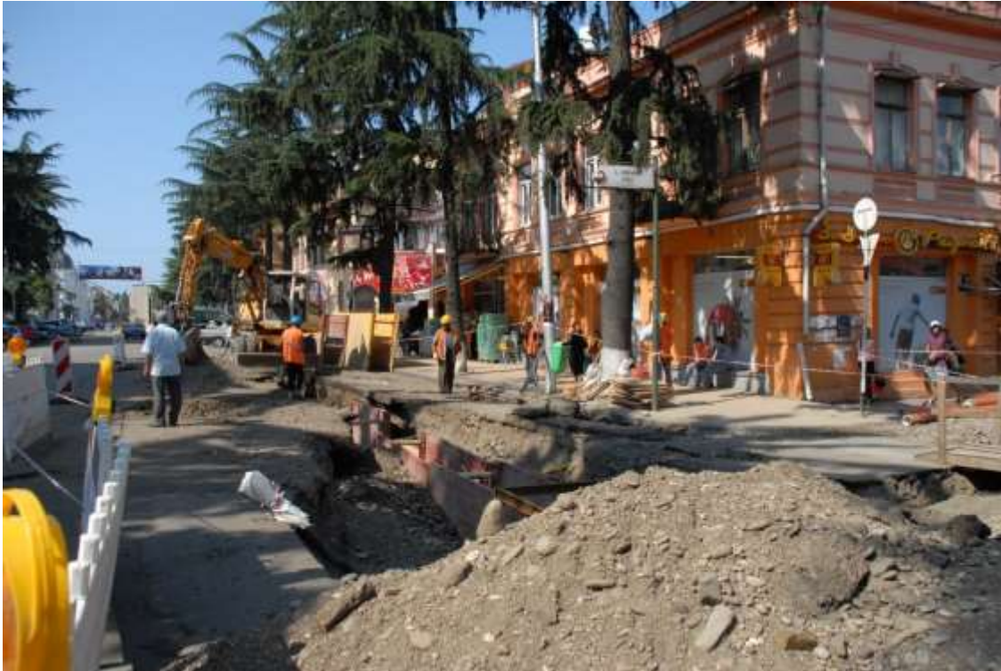
Picture 2 Rehabilitation process of one of the streets
