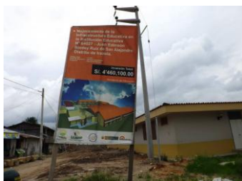
Figure 18: Renovation of the school (Facebook, 2014)
