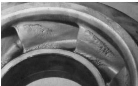
Figure 1-3. Cavitation erosion in a centrifugal pump impeller.
