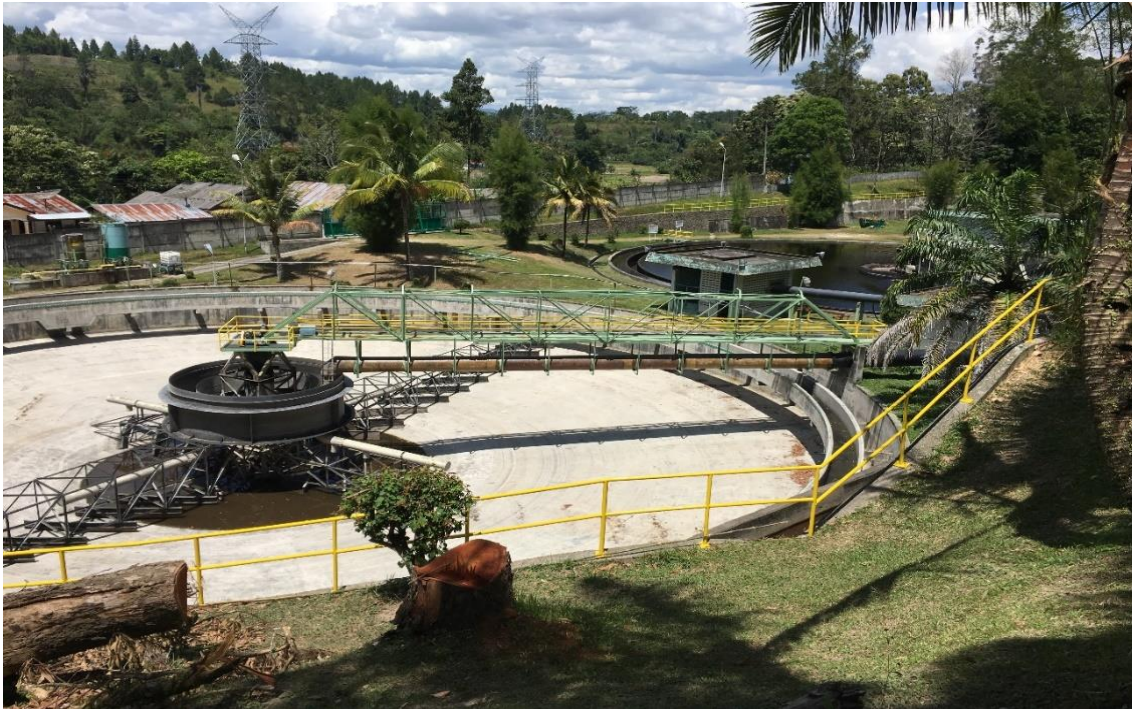
Appendix 3: TPL's wastewater treatment tank (Author 2018).
