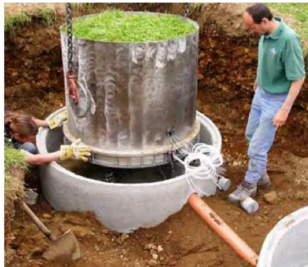
Obr. 3.23: Instalace Hydro-Lyzimetru [27]
