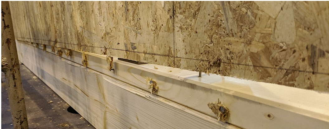
Figure 5.7 – Progressive failure of sheathing-to-framing fasteners in bottom rail
