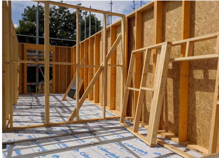
Figure 1.1 – Open panel timber frame [1]
