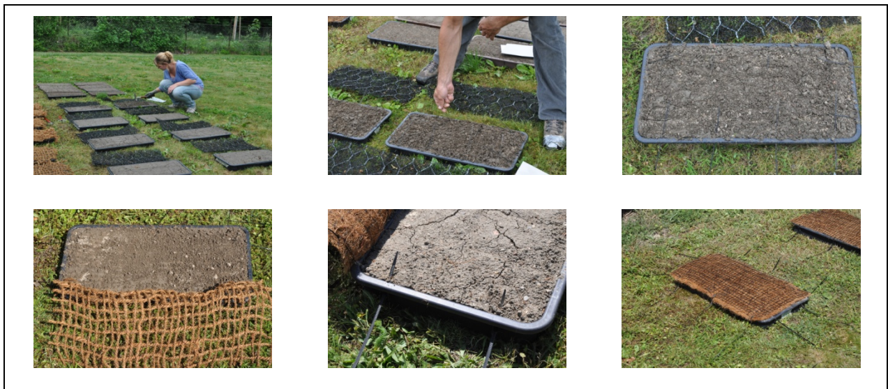
Figure 15 Sowing and installation of geotextiles (18.05.2012, 22.05.2012 Essling, VIENNA)
