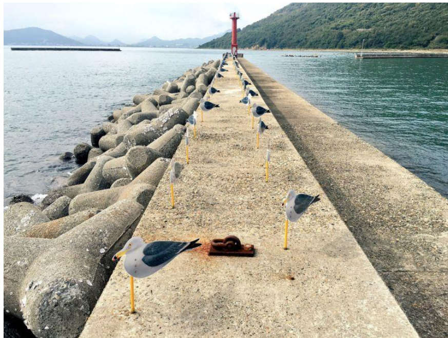
Figure 26— Japanese sea barrier with tetrapods (arstechnica.com)
