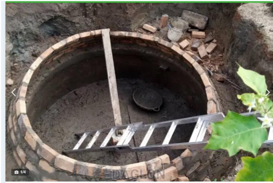
Figure 9: A biogas digester under construction in Ghana (source: Taken online from DAGLON-TECH, Ghana).
