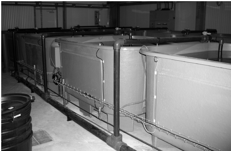
Fig. 4. Suitable recirculating aquaculture system used for intensive culture of older pikeperch, Sander lucioperca (L.) in Asialor Ltd. company, France (photo T. Policar).
