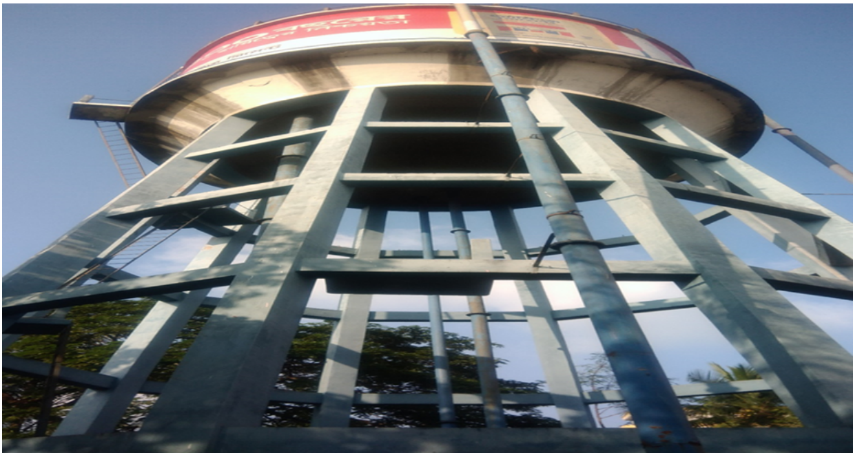
Figure 12: The main water tower (reservoir) of untreated water (water is supply from the local water wells)
