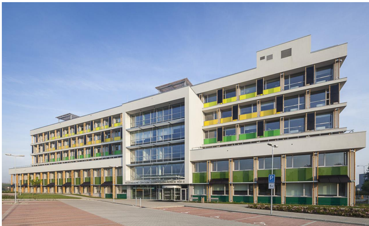
Obr. 7 Jižní pohled na budovu MCEV II (dostupné z: < https://www.archdesign.cz/en/projekty/education/czech-university-of-life-sciences-prague-cross-faculty-centre-for-environmental-sciences-phase-ii/ >)
