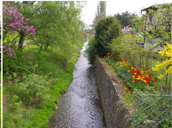
Figure 19: The concrete wall in summer house area
