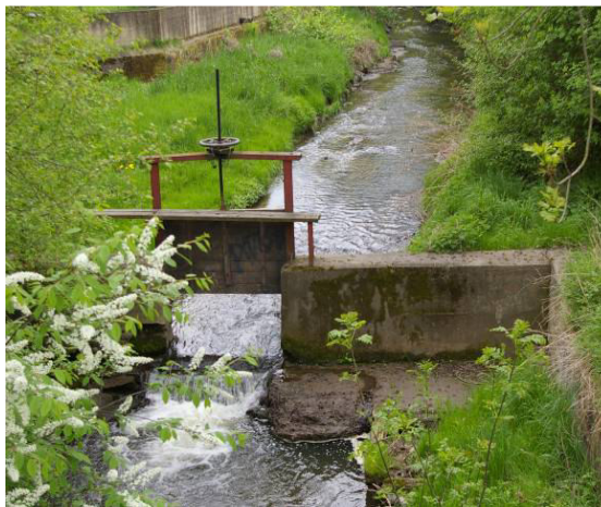
Figure 32: Weir with water gate after the canalization
