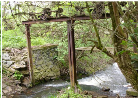
Figure 40: Old weir with water gate – the iron structure
