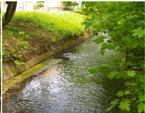
Figure 21: A concrete channel in Olovnice village
