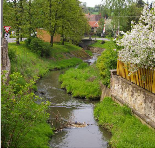
Figure 23: Concrete channel in Olovnice village
