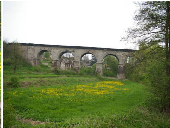
Figure 38: Viaduct away the village Podlešín
